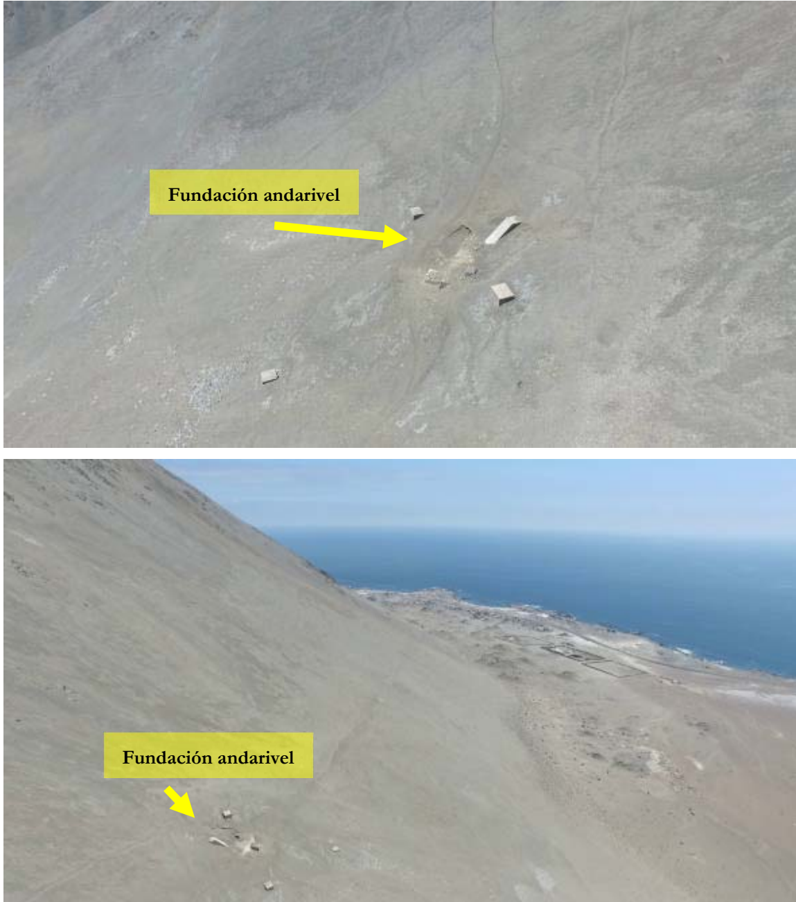
Figure 6-5 Aerial view of the foundations of the lift (VE-31)
