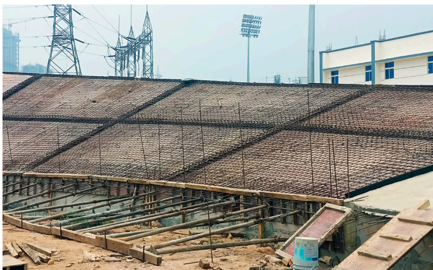
Reinforced Cement Concrete (RCC) work being carried out during the construction of the cycling velodrome
